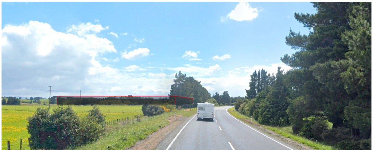
Figure 3 – View from SH6 toward the Terminal Substation
